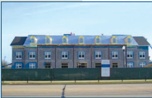
The front of the chapter house is beginning to take shape.
